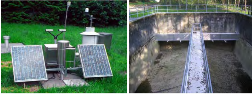
Fig. 1. Left: rain gauge (pluviometer). Right: stormwater tank.
